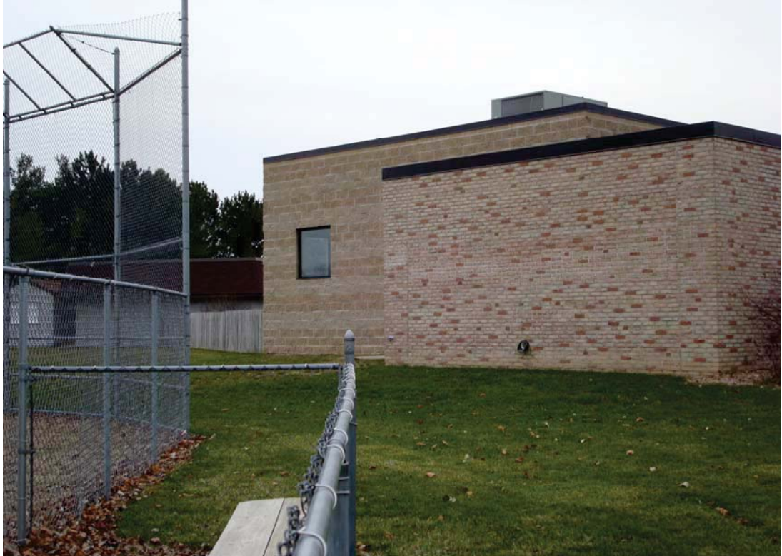
- Wall where scoreboard is to be installed.
