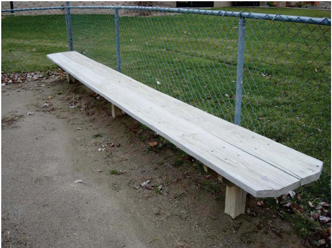
- Dugout Benches before, screws sticking up and splinters
