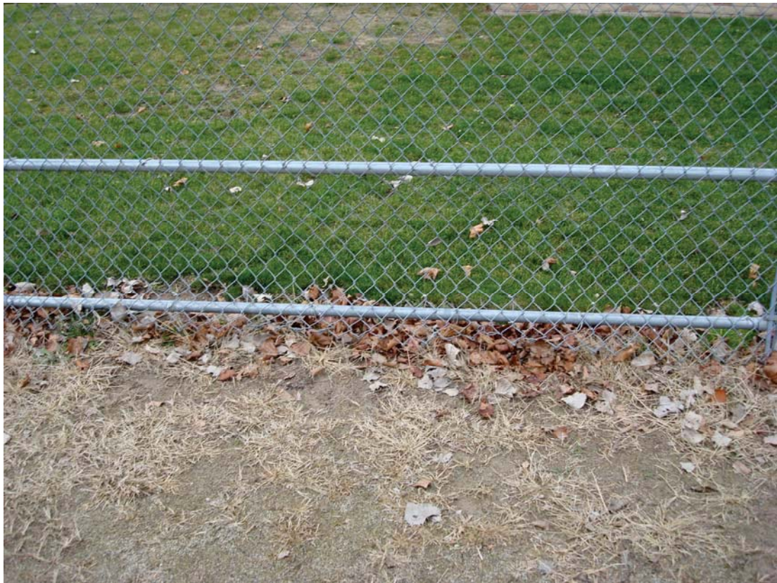
- Backstop before 2x6 stopper installation. More crabgrass to be removed.
